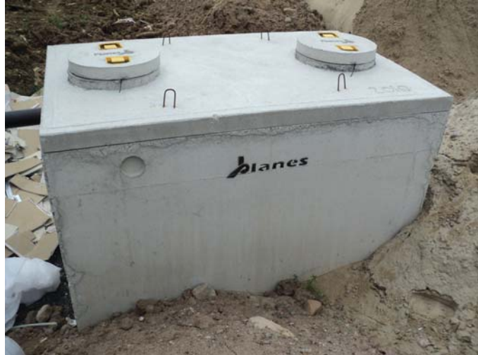
A septic tank (shown above) and tile bed are the main components of most on-site sewage or septic systems.
