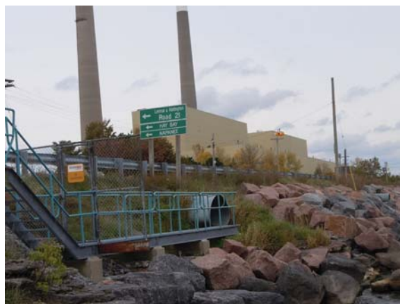
The A.L. Dafoe (Greater Napanee) intake with Highway 33 and Lennox Generating Station in the background.
